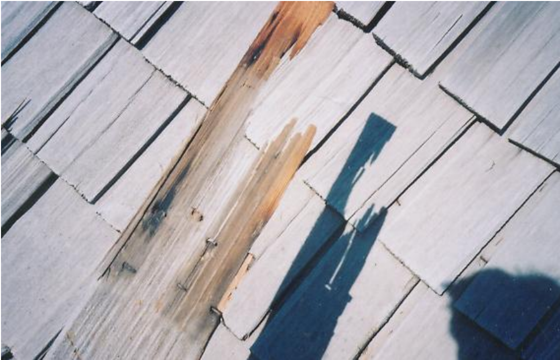
Close-up of a burned out shingle. Notice the shadow. Lovely, isn't it?
