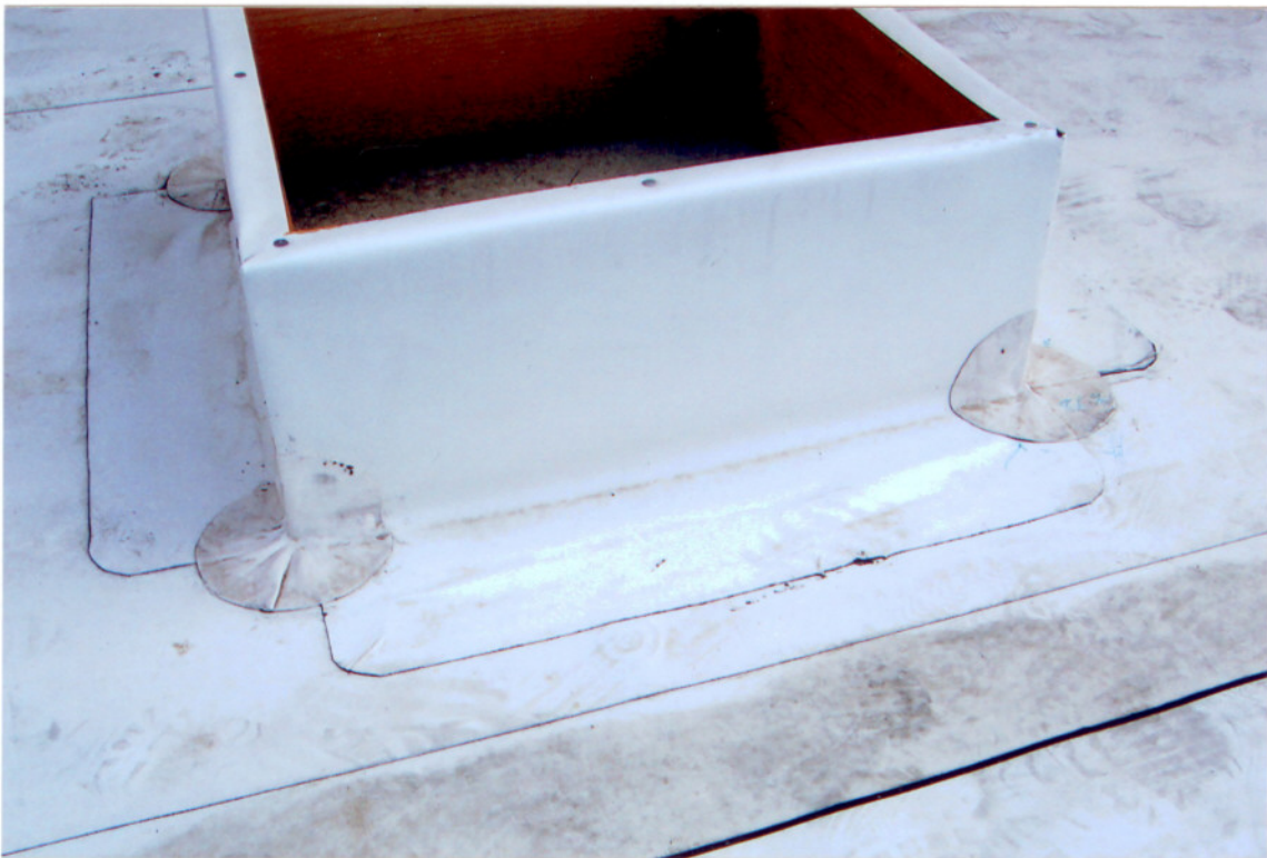
Picture #14 A properly flashed skylight.
