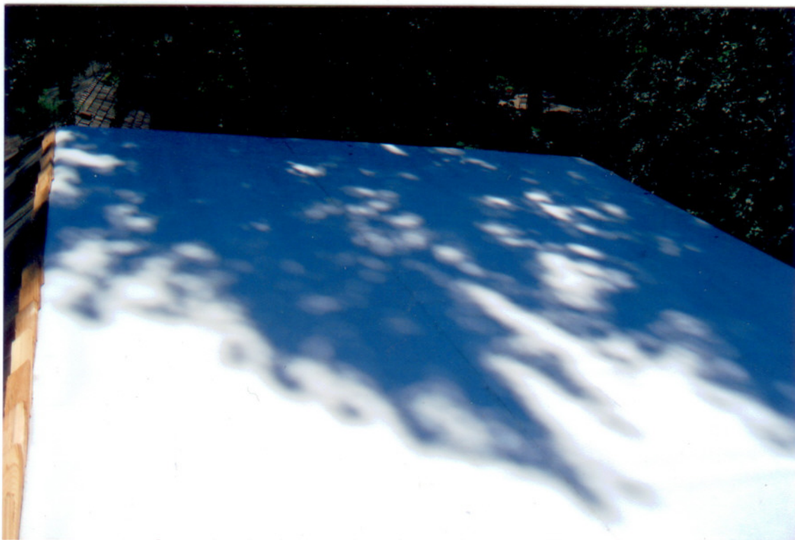
Picture #2 Many of the TPO flatroofs we install on homes are bump-out dormers.
