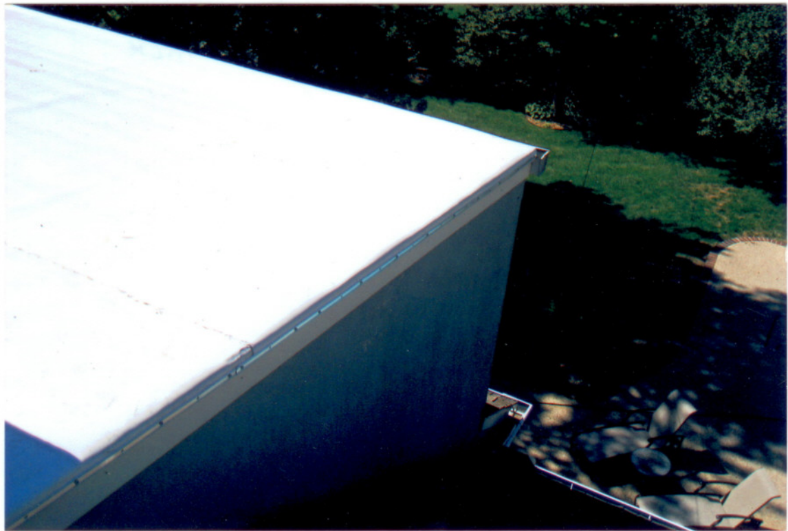
Picture #4 Detail of a dormer flatroof.
