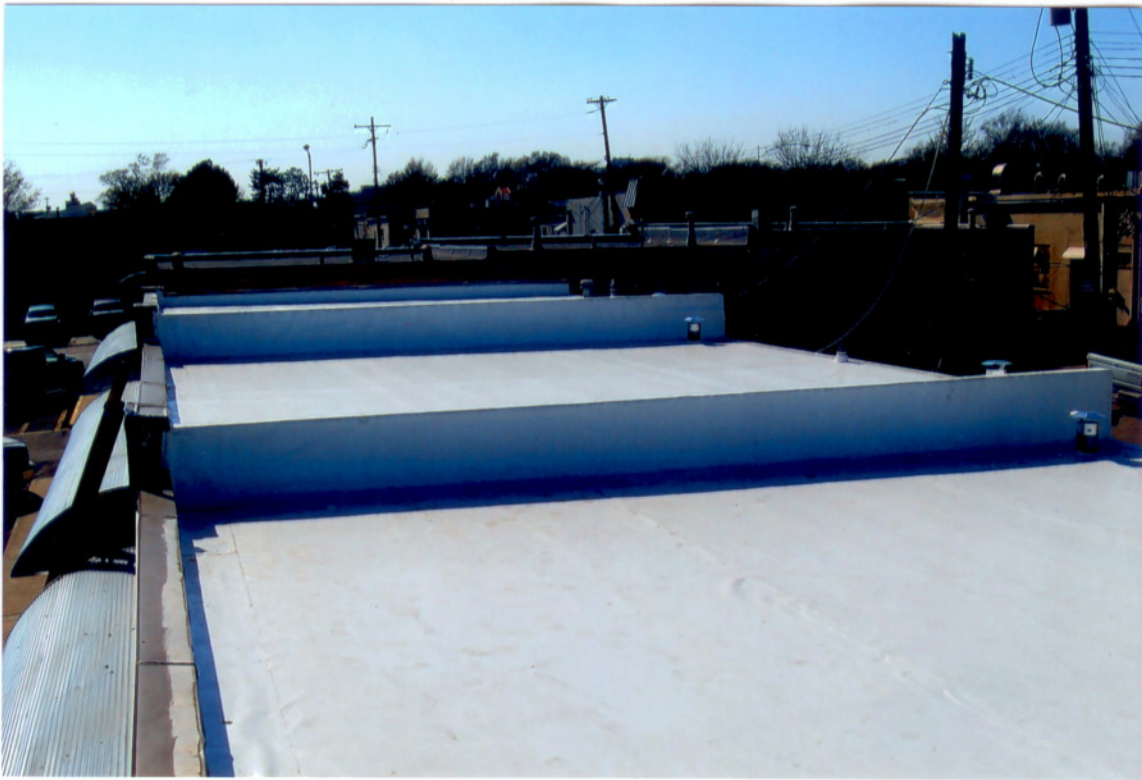
Picture #18 TPO was the perfect product for this strip mall.
