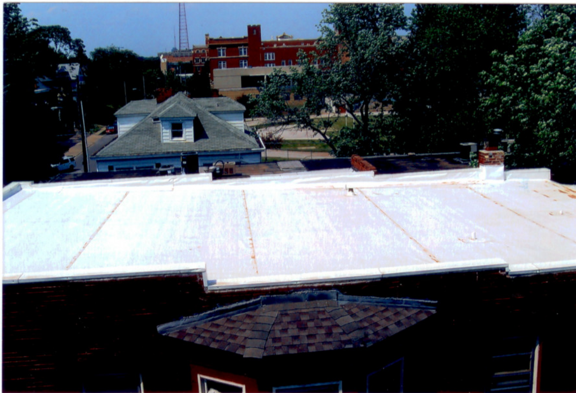
Picture #21 If necessary, we can custom construct new parapet caps.
