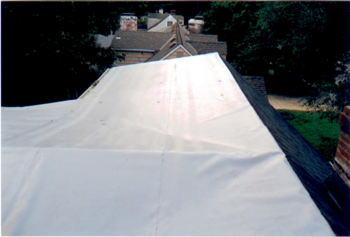
Picture #7 TPO roofs conform well to uneven roof planes.
