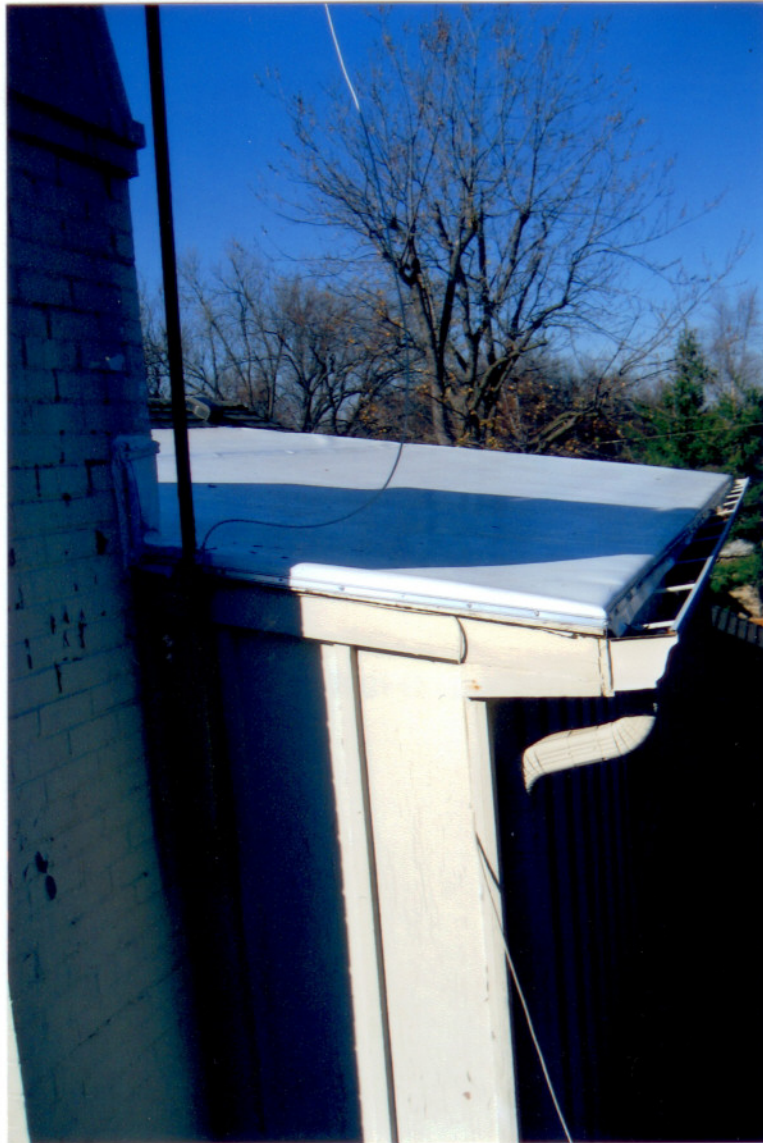
Picture #5 Another TPO roof on a dormer flatroof.
