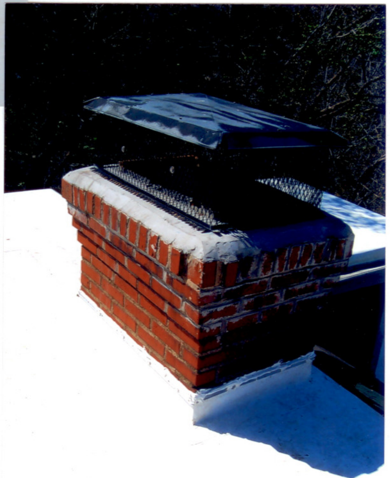
Picture #12 We can properly flash a chimney, even on a flatroof.
