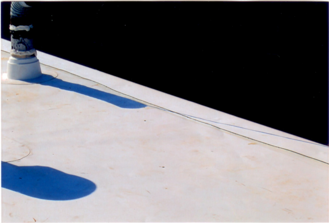
Picture #16 The amount of water caught against the backseam of the seal-down strip is negligible.
