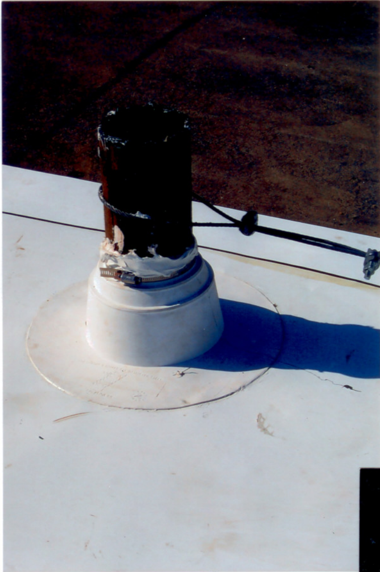
Picture #11 Plumbing pipe flashing detail.
