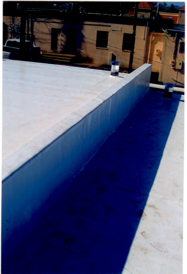
Picture #19 TPO remains pliable long after installation, so it will not tear or crack when stretched over parapet walls.
