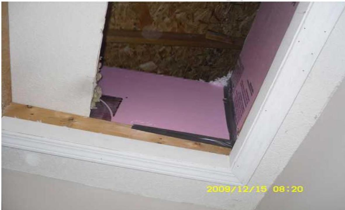
(above) Pink rigid insulation board creates a barrier to keep attic insulation from just flopping down into your living area.
