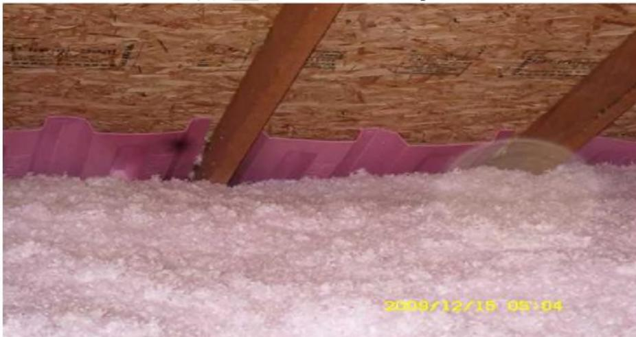
**ATTIC RAFTER BAFFLES** (The darker pink rigid Styrofoam directly against the underside of the plywood). Baffles allow air to flow directly under the plywood even when the insulation is filled tight into the corners of the roof.
