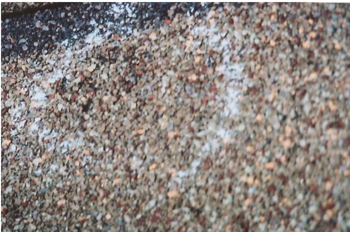
Photo #5 Hail hits on composition shingle.
