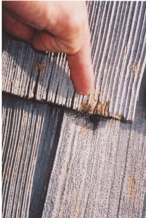
Photo #9 Butt rot hits still count if fresh wood is exposed.
