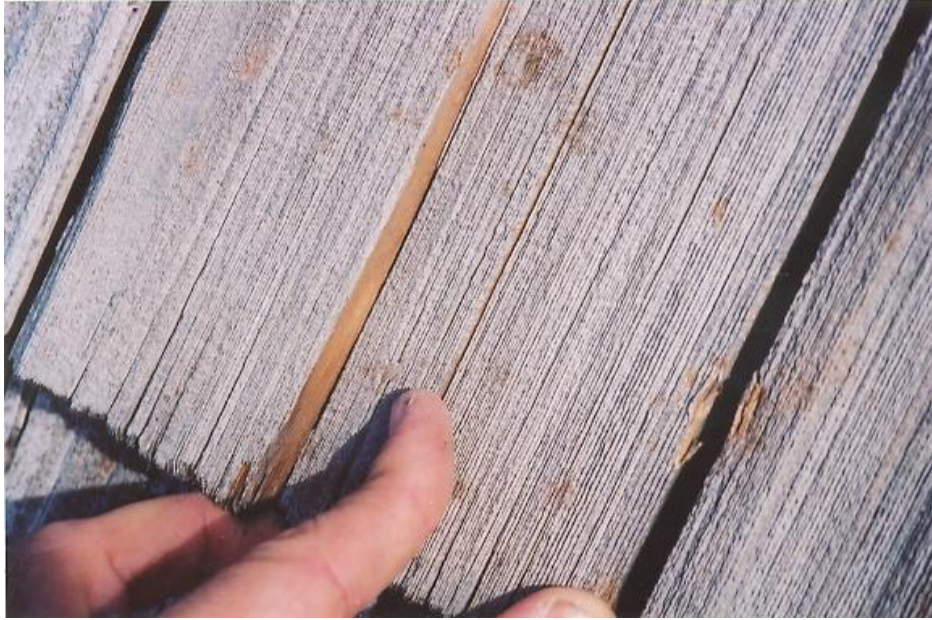
Multiple hits and cracks on the same shingle count as multiple hits per HAAG
