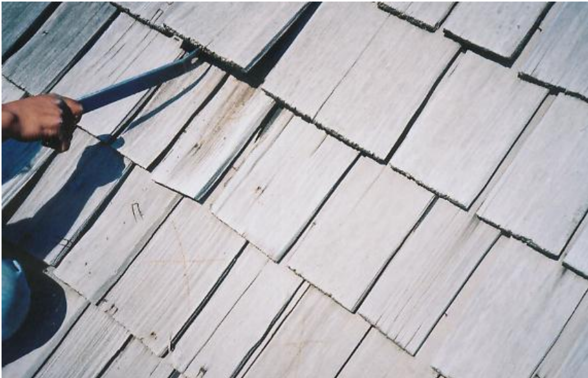
Removing fasteners
