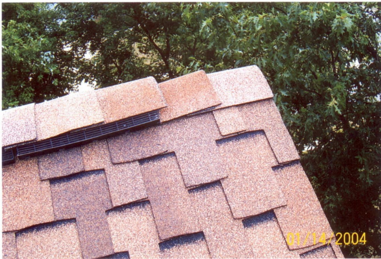
**Ridge Vent # 3. Ridge vents should end about 1 foot away from the end gable (more with open soffits).**
