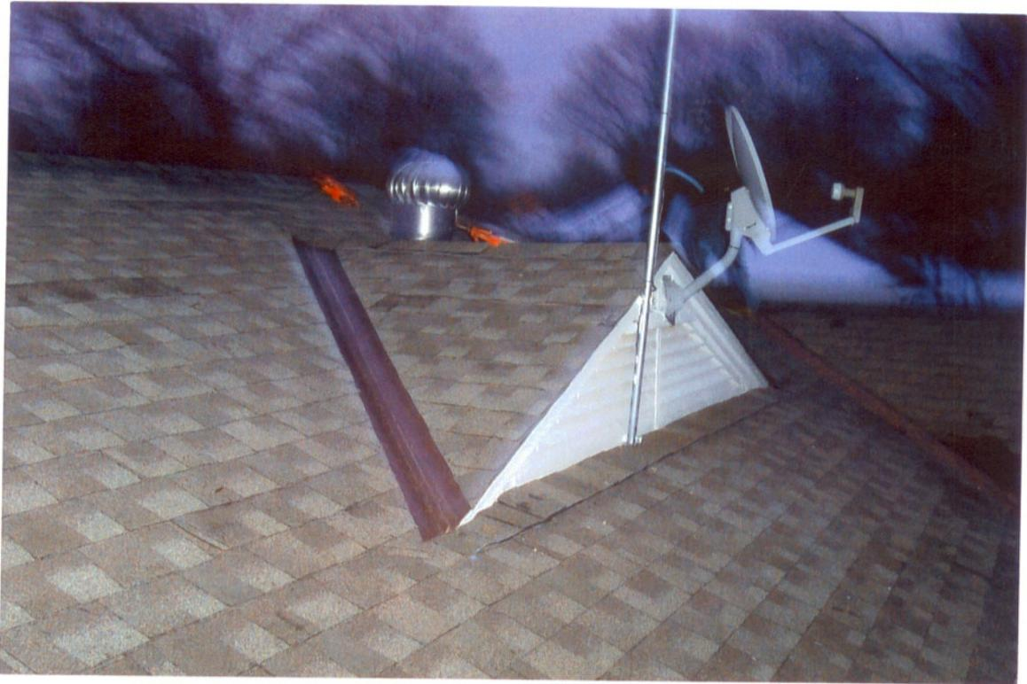
**Dormer Vent. We will sometimes remove dormer vents like this, and simply roof over the area.**
