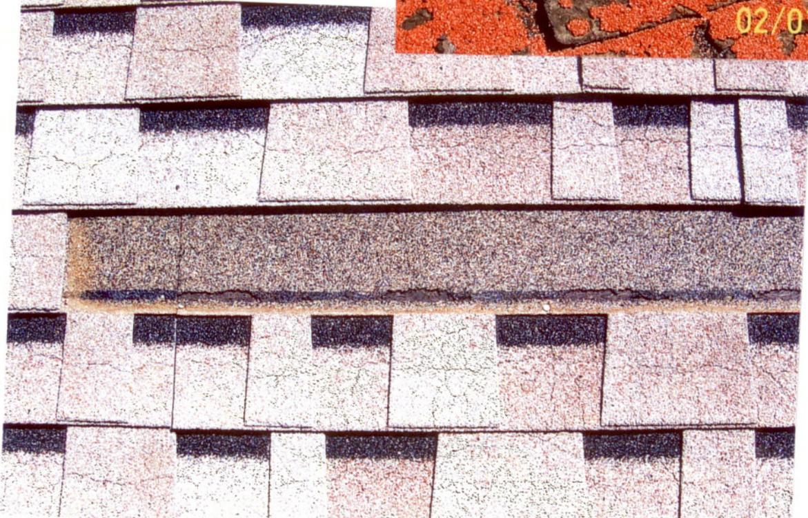
Sometimes heat-damaged shingles will have long cracks in the shingles surface, called “Crazing”
